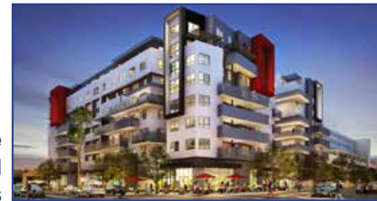
Secure Personnel & Facilities
